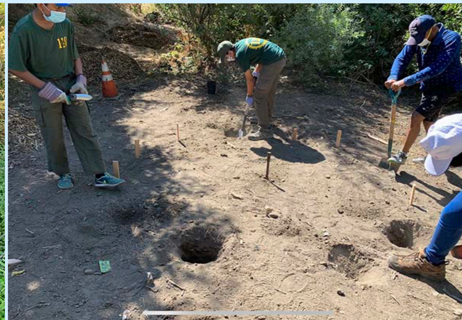
making holes for support
