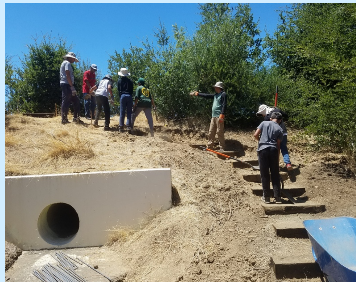
putting in stairs and trail
